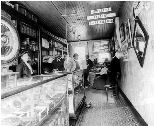
Interior of African-American store.
